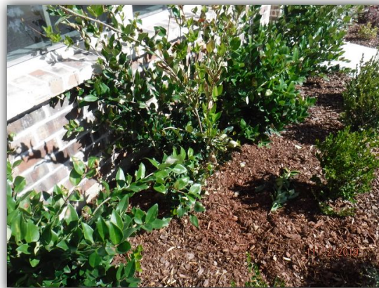
Bushes planted too close to walls at front of house. Vegetation should be kept at least 12 inches from a wall
