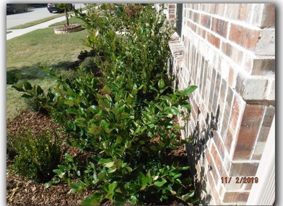
Bushes planted too close to walls at front of house. Vegetation should be kept at least 12 inches from a wall
