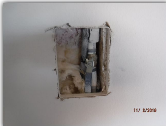
No cover on main water shutoff on garage back wall
