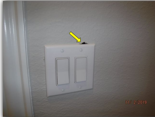
There is a hole above the electrical plate in the master bath
