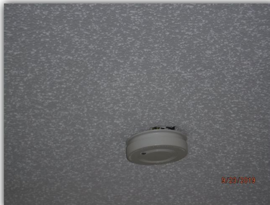
The smoke alarm in the front office is chirping due to low battery
