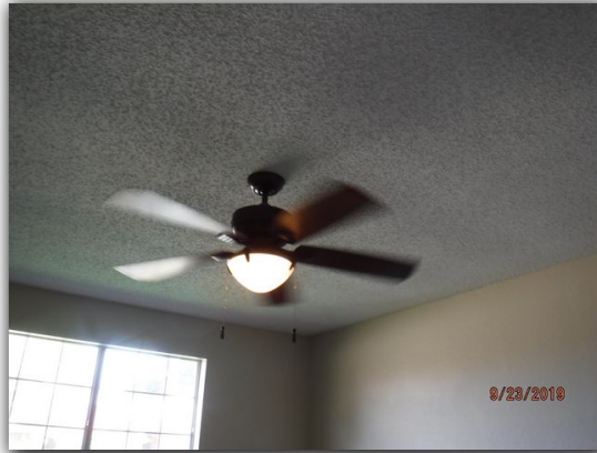
The outlet for the microwave has no cover
