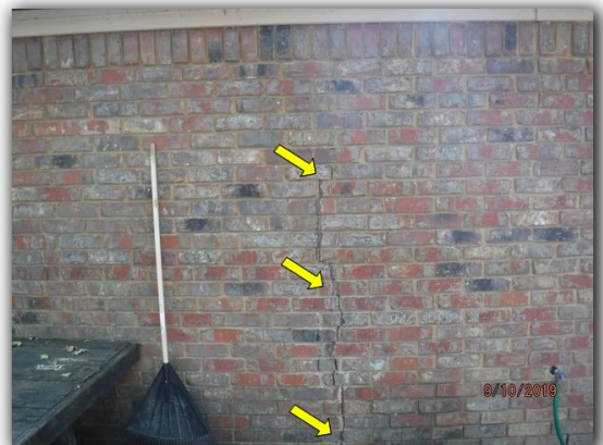
West wall serving the master bedroom has a 1/4 inch crack from upper portion of wall to foundation.
