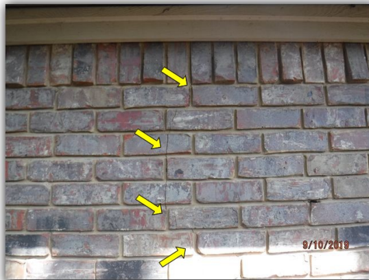
West wall serving the master bedroom has a 1/4 inch crack from upper portion of wall to foundation.
