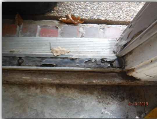
The garage side entry door has rotted wood at the bottom and rotted threshold weather stripping
