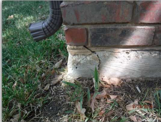
South wall foundation has two hairline cracks
