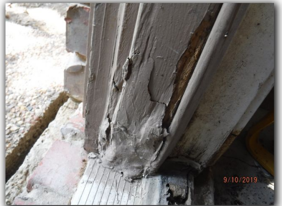
The garage side entry door has rotted wood at the bottom and rotted threshold weather stripping
