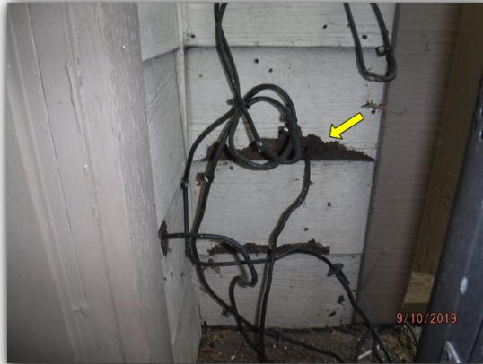
The front porch has rotted siding at the bottom of the wall. It also has two holes in the wall
