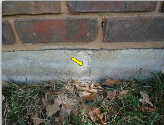
Corner pop on south wall about midway the wall
