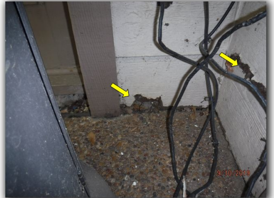
The front porch has rotted siding at the bottom of the wall. It also has two holes in the wall
