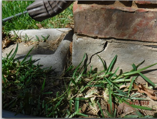
Corner pop on south wall near the AC unit
