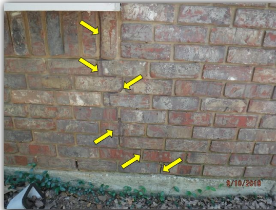
1/8 inch crack from corner of kitchen window to slab
